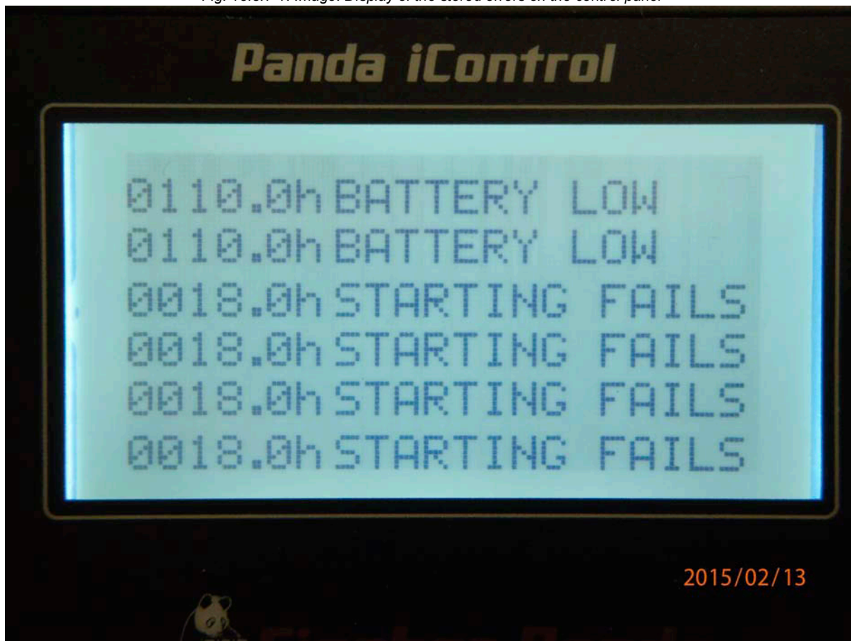
Fig. 18.3.7-1: Image: Display of the stored errors on the control panel
